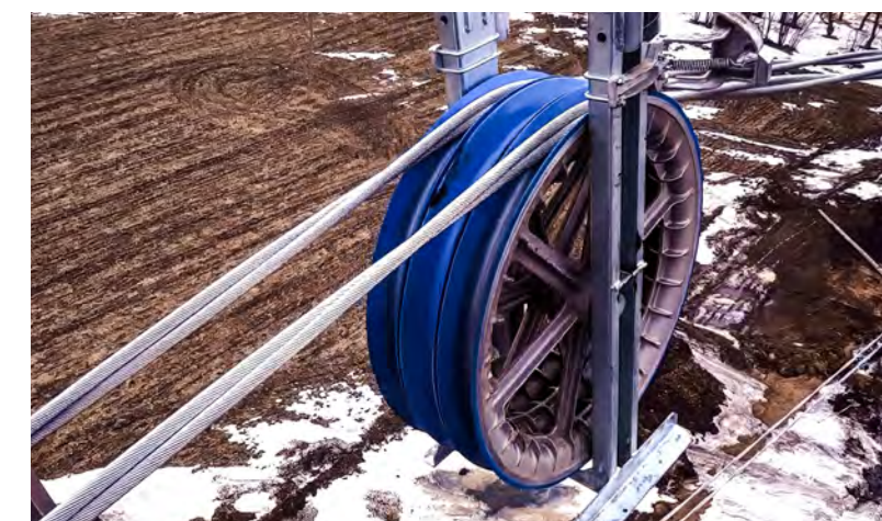
Specialty bundle block sheave groove for twisted pair conductor
